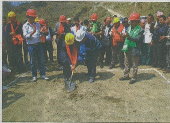
Workers preparing to lay the foundation stone of Nyadi Hydropower Project, in Lamjung, on Friday.
